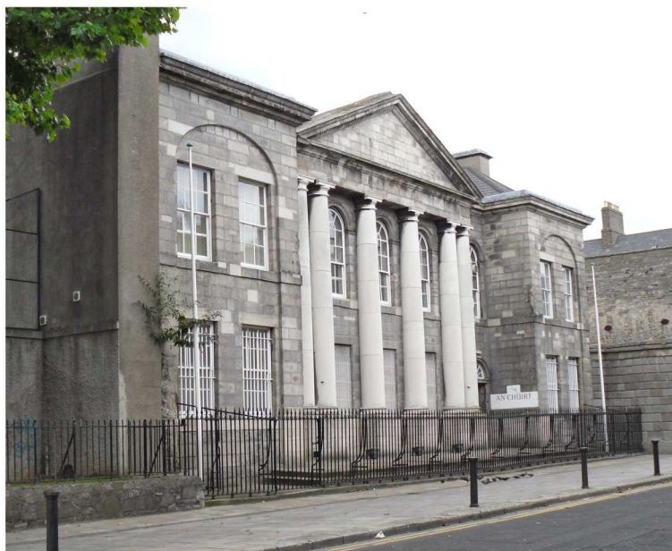
Fig 1.7 Green Street Courthouse, Dublin. At the time of this picture (July 2011) restoration work was under way and so no photography of the interior was possible. The building is very close to North Anne Street and it would have been only a short walk for WGG from his home to attend the court for jury service.
