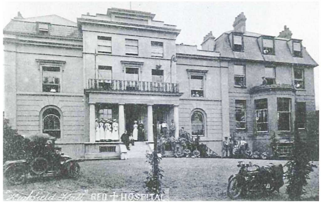
Fig 8.13 This is almost certainly the building previously known as Highfield Mansions, which was the home of Augusta Jenkins and her daughter in 1907. (It later became a hospital and was demolished in 1932 27 .)
